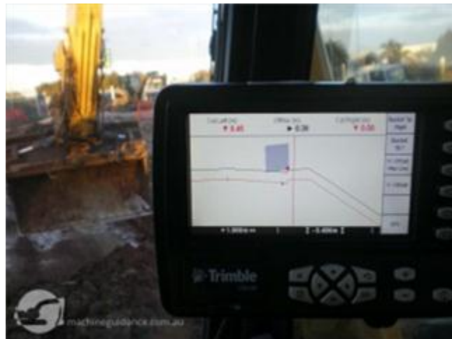
Figure 5 3D Machine Guidance Interface setup on excavator
